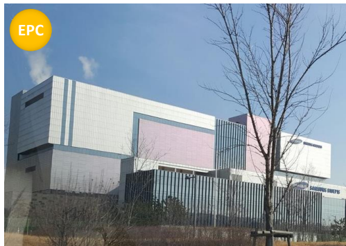
SBL BIO CDMO#1 증축 Project
